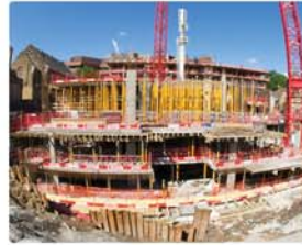
Extensive Double Basement and Podium Slab..
