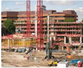
Design and Build for the construction of two blocks.
