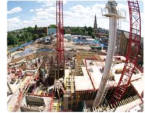
Completed on a tight, city centre site in Ealing.
