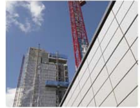
Also includes, 4900m2 of Cat A Office fit-out.
