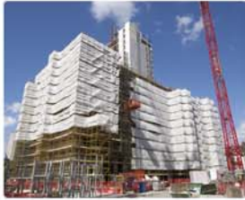
Design and Build for the delivery of 445 units.
