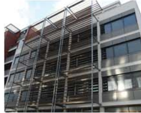
Bespoke galvanised balconies, metalwork and louvers.
