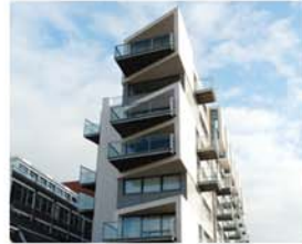
Works included new build and refurbishment.
