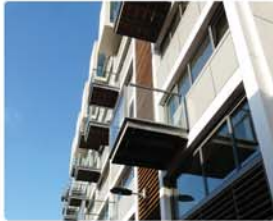
63 work/live units - duplex apartments.
